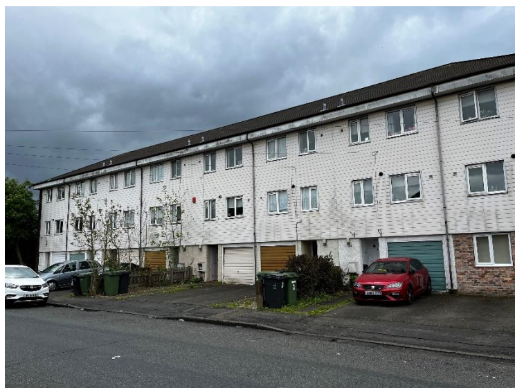
The three-storey Wolverhampton Wimpey No-Fines houses before surveying
