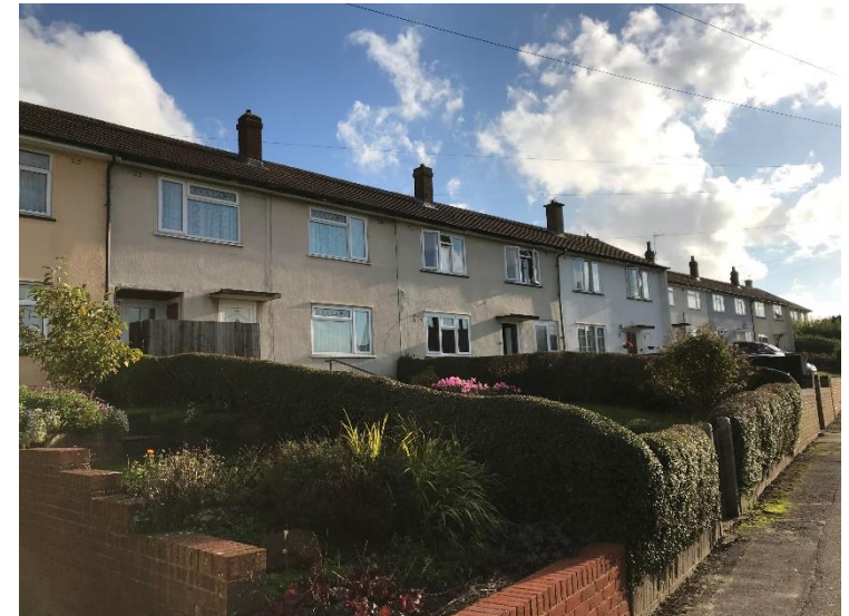
A typical street scene of solid wall Laing Easiform archetypal homes in Kent
